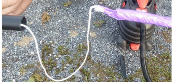
Figure 7: The kite string taped to the rope with a "point" to guide the rope through the tubing
